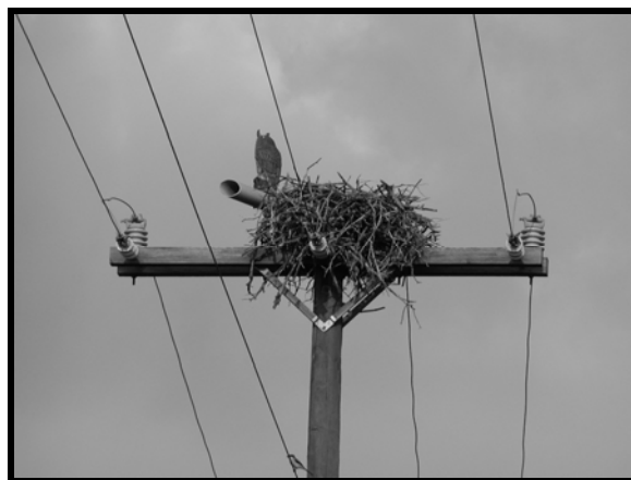
Photo 8 Osprey Nest on Double Deadend Unit with an Ineffective Stick Deflector and Owl Effigy
