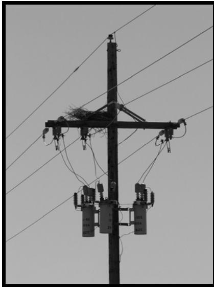
Photo 2 Distribution Recloser Pole with an Active Red-tailed Hawk Nest on Double Crossarms
